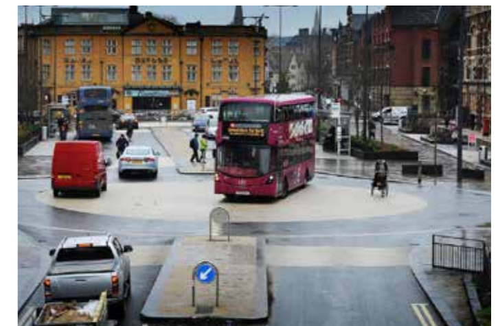
Example of alternative junction design in a slow traffic environment (Frideswide Square, Oxford)
