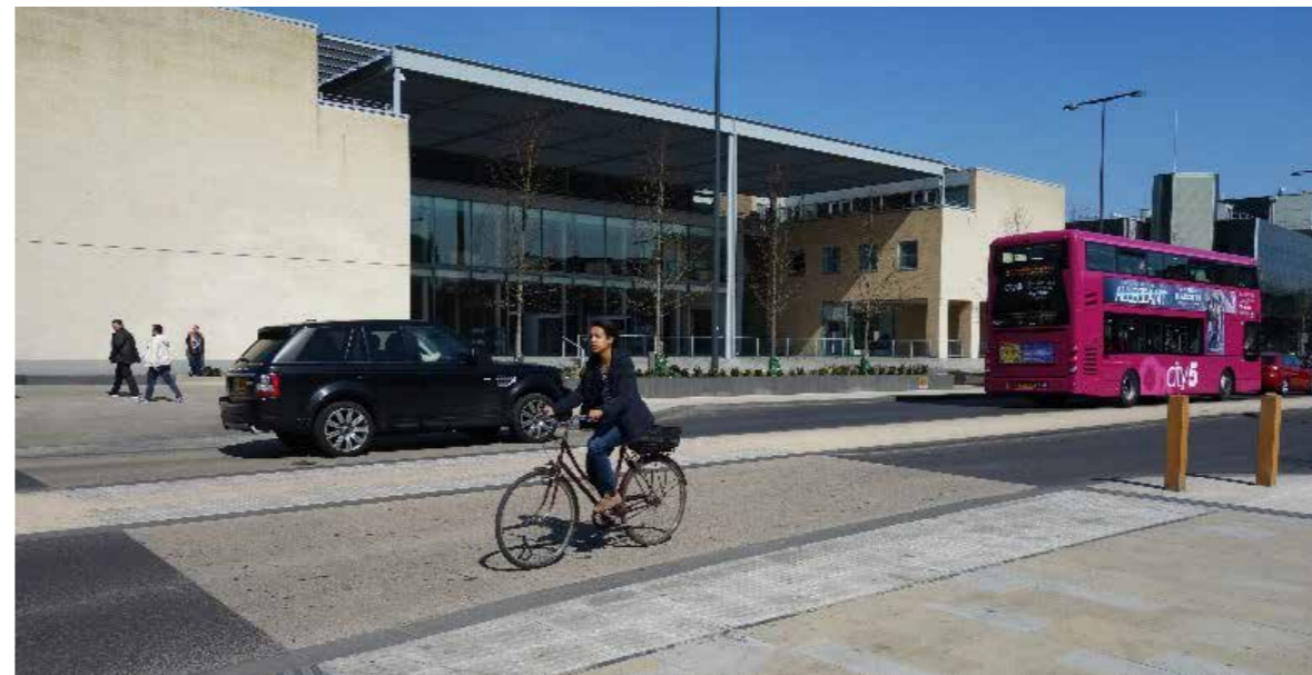
Example of gateway area with central median, special carriageway surfacing, and pedestrian crossing (Frideswide Square, Oxford)
