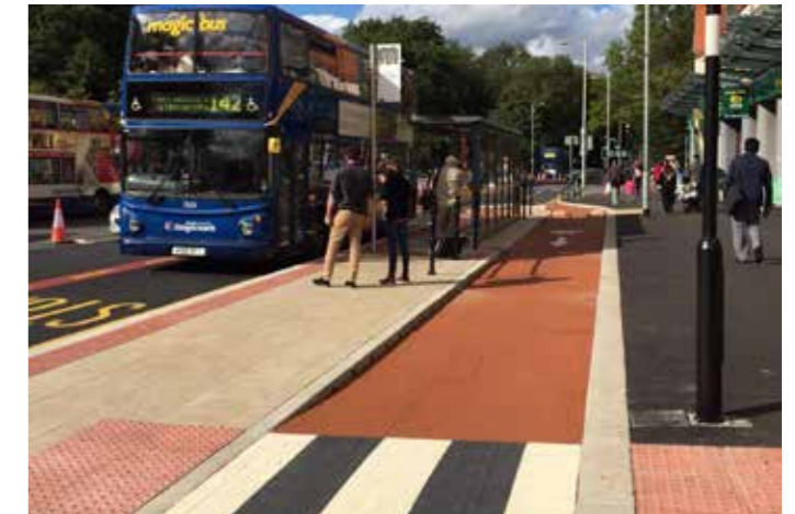
Example of cycle lane and 'floating' bus stop (Oxford Road, Manchester)
