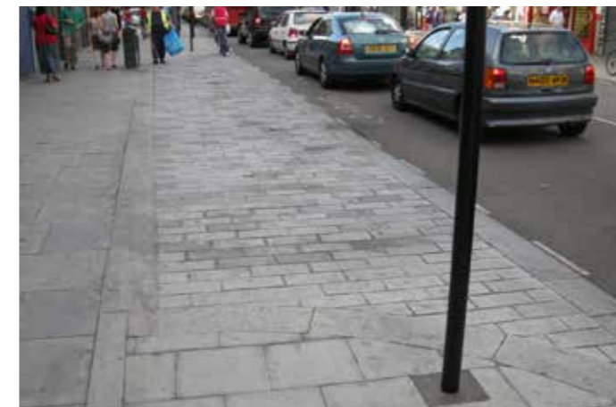
Example of loading bay integrated within the footway (Walworth Road, London)
