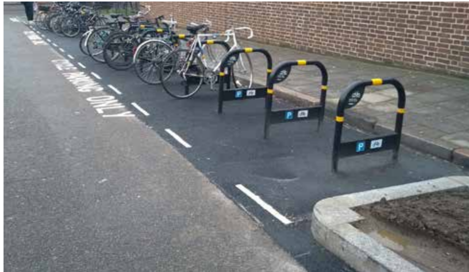
Examples of cycle parking in a re-purposed car parking space, installed in with footway build-outs at each end (Hackney, London)
