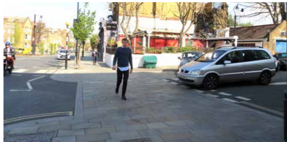
Examples of continuous footway crossing providing level surface and pedestrian priority over a side road entry (from top: Greenwich; Southall; and Clapham, London)
