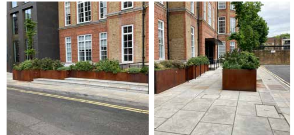
Planters used as both retaining wall and to reduce amount of railings for level change
