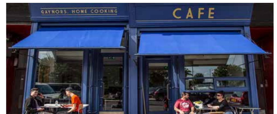
Examples of the results of shop front and facade improvement schemes: top, Leyton, London; bottom, Glasgow.
